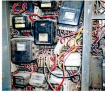
Fig. 4.27 Poor and Shabby Meter
