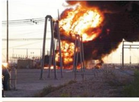
fig. 2.35 Transformer Fire Due to Overload
