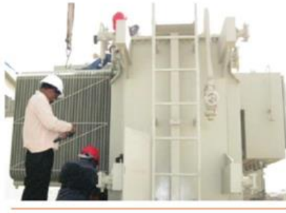
Fig. 2.36 Maintenance of Transformer on Site
