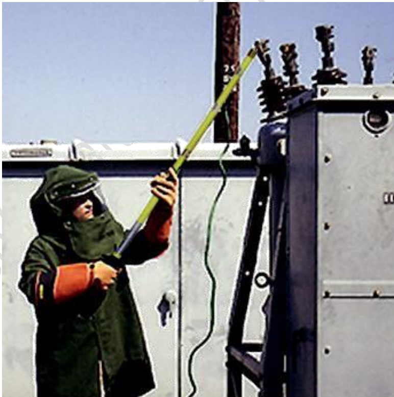
Fig. 4.8 Working with Discharge Rod
