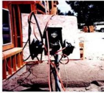
Fig. 4.28 Too Many Circuits are Open
