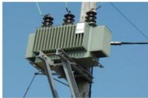
Fig. 2.4 Pole Mounted Transformer
